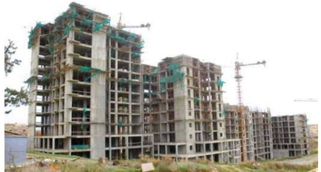
Housing Construction in Algiers
